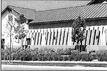
3.2.2.7 b) Low rise, landscaped screening walls contribute to a more attractive environment.
